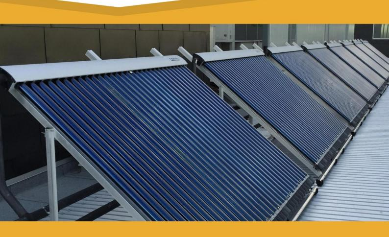
CONSOL 30-58-1800 COLLECTOR FLAT MOUNT ON METAL TILE ROOF VALVE VENT, OPEN LOOP
