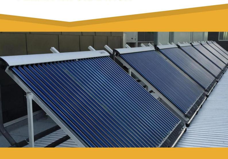
CONSOL 30-58-1800 COLLECTOR FRAME MOUNT ON BUTYNOL ROOF VALVE VENT, OPEN LOOP
