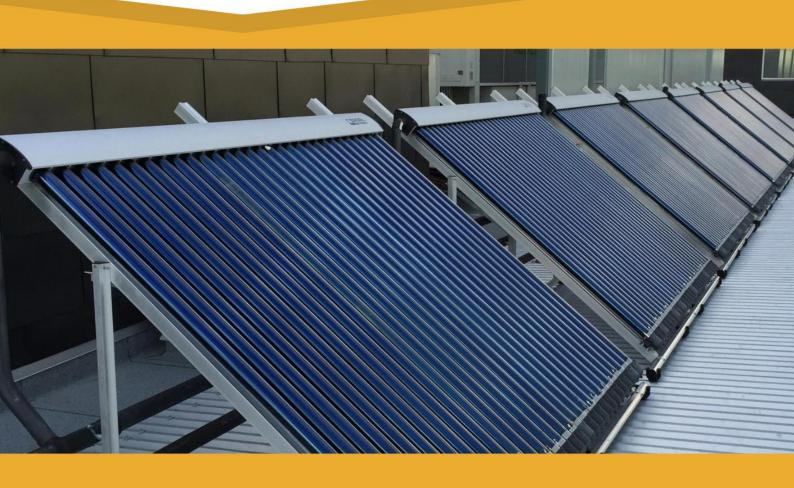
CONSOL 30-58-1800 COLLECTOR FRAME MOUNT ON CORRUGATE IRON ROOF VALVE VENT, OPEN LOOP
